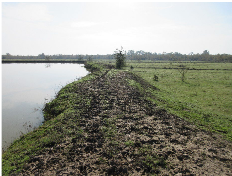
Fig. 11. Site LS089: View of the water reservoir facing east.
