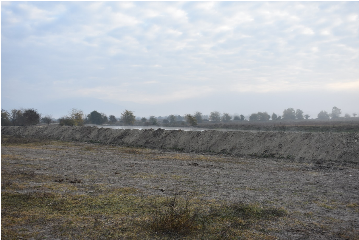
Fig. 3. View of site LS071 facing NE.
